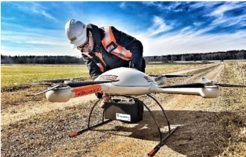
Figure 7 – Data acquisition by drone on the construction of R2 Kriváň - Mýtňa
